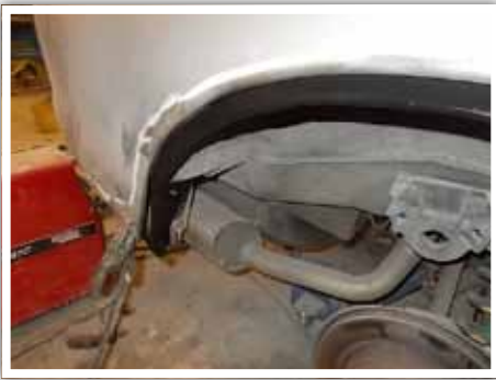
One of the new wheelarch lip repair panel in place.
